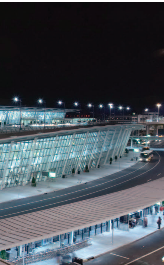
Direct involvement of political leaders and management staff effectively facilitated the redevelopment of the JFK Terminal 4 Gateway.
